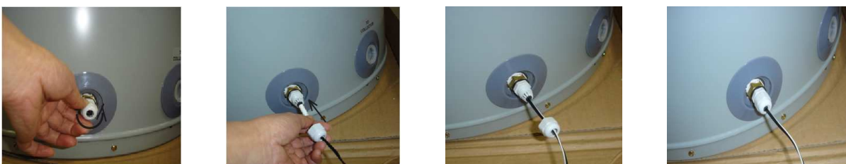
Example of sensor installation.
